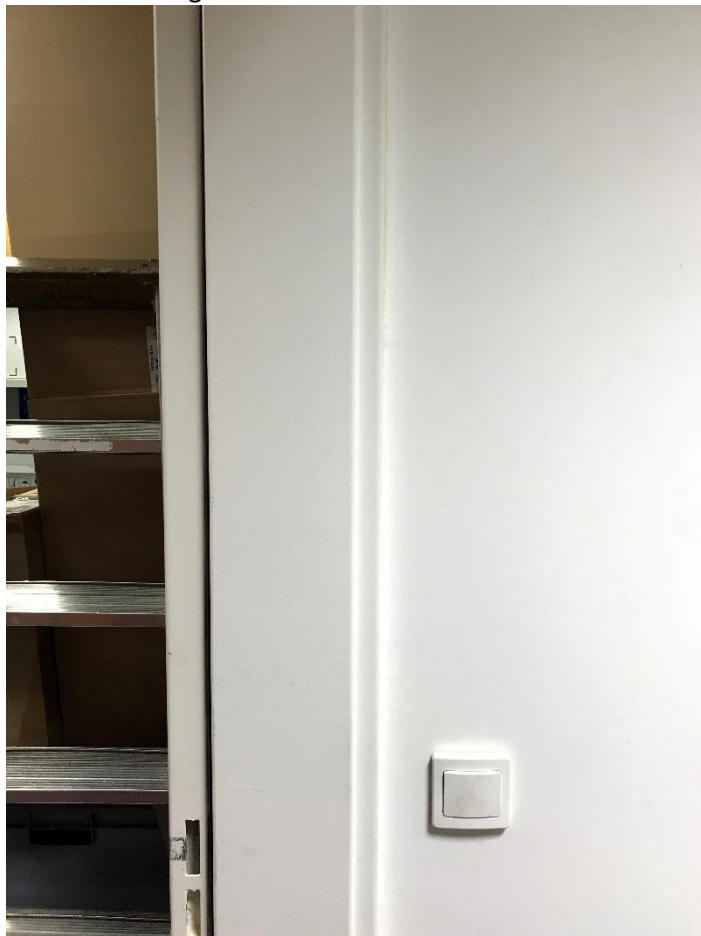
Photo 2 - through the tech room door
