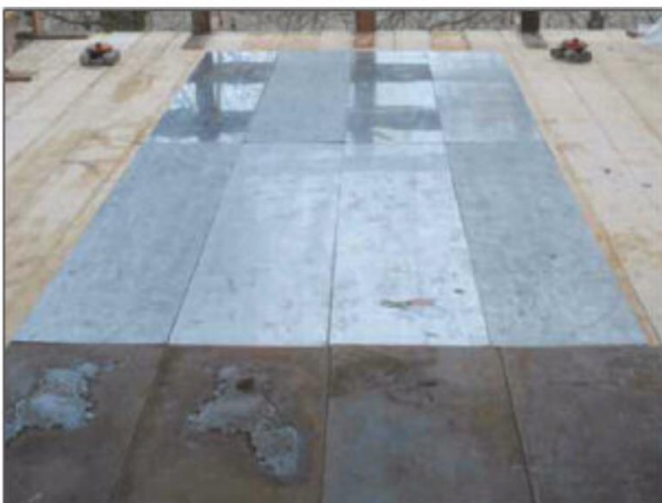
Fig. 21 Positioning the steel plates
