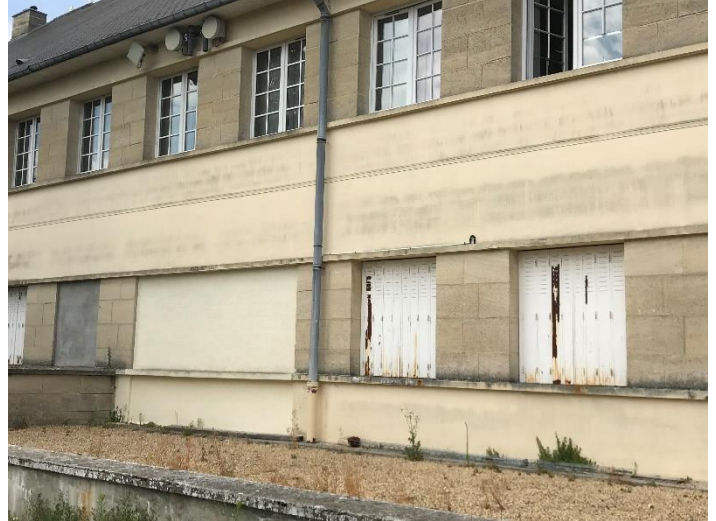
Photo 9 – RF wall opening
